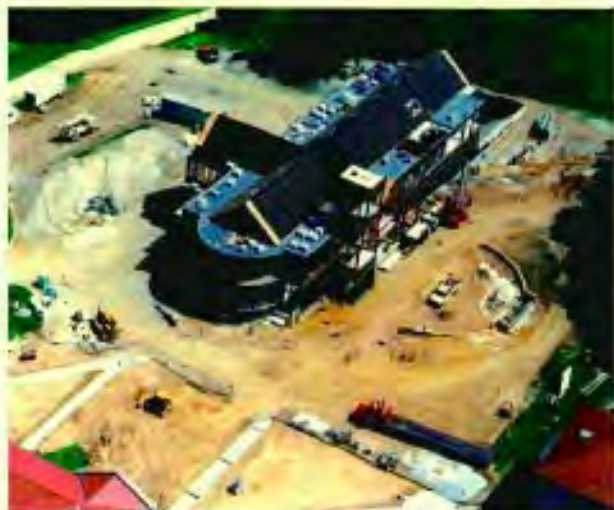
Early stage of work. Photo by Rick Sencora
